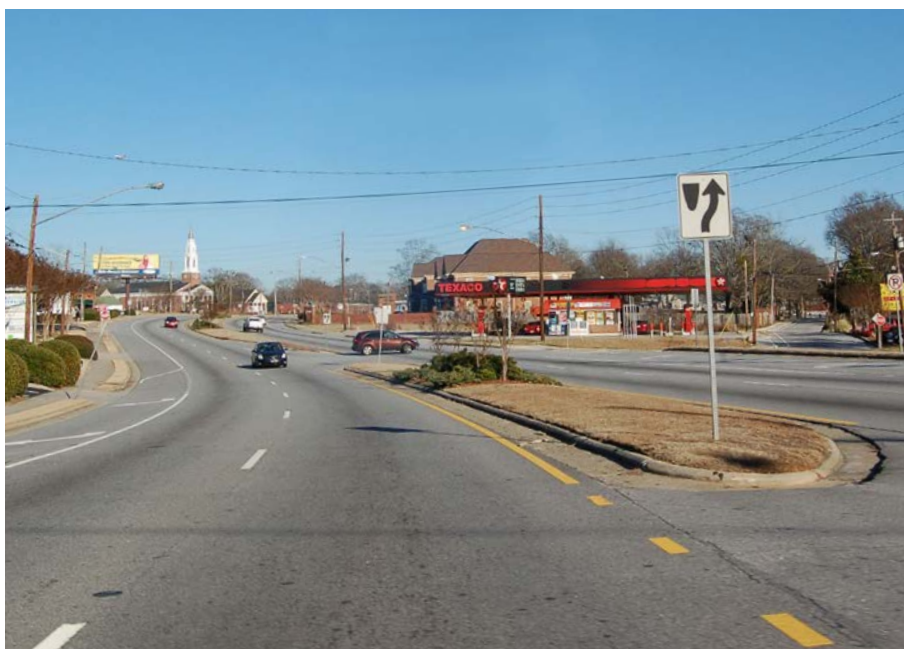
Roads designed for high-speed traffic were identified as barriers to walking and biking by forum participants.
