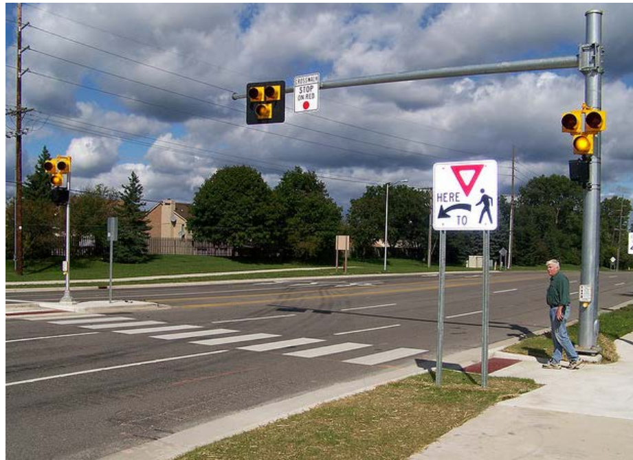
Accessible push buttons, textured curb ramps, signalized crossings, and high visibility cross walks improve crossing safety for all users."
