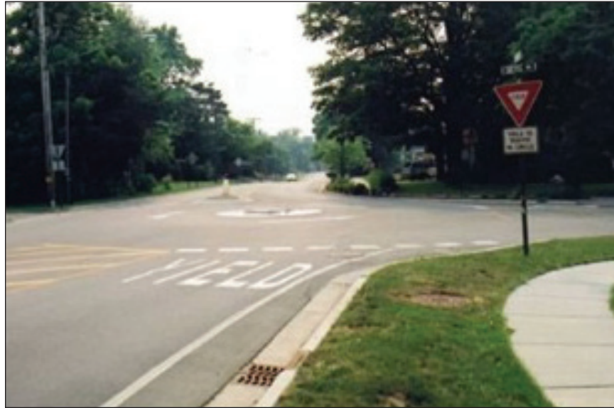
Figure 38: Traversable Island Construction
