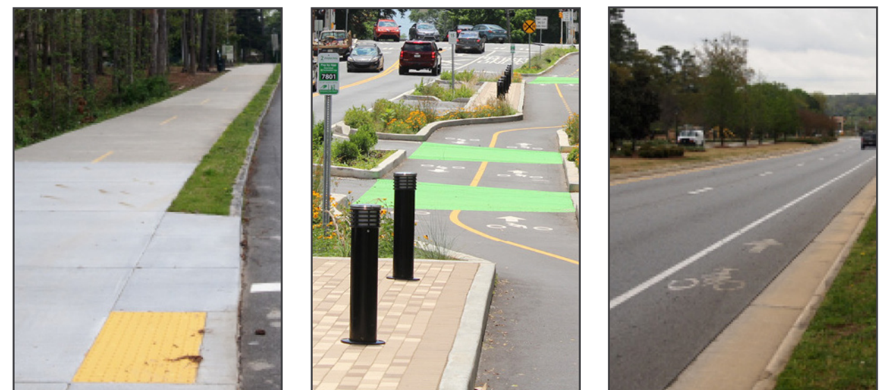
Bikeway facility types vary widely across the metro Atlanta region. ARC's 2019 bicycle facility inventory includes three broad categories: multi-use paths; separated (or protected) bike lanes; and painted bike lanes. From left to right: Barclay Dr, Dunwoody; Abernathy Blvd, Sandy Springs; McDonough St, Decatur. Source: ARC.
