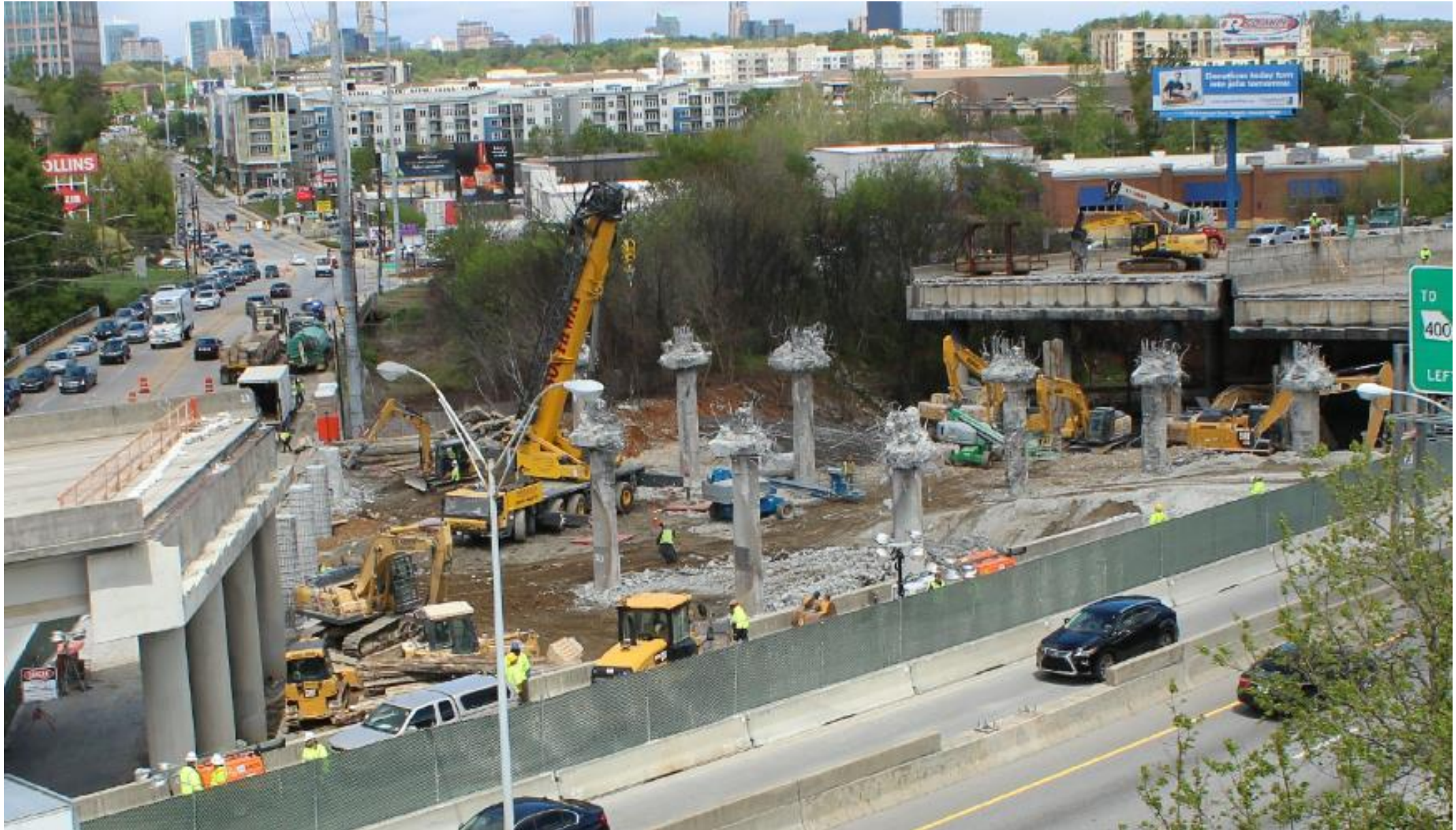
Interstate 85 Bridge Rebuild – Thursday afternoon, April 6, 2017
