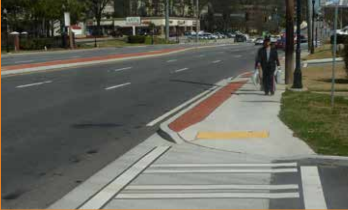
Basic sidewalk infrastructure on major road
