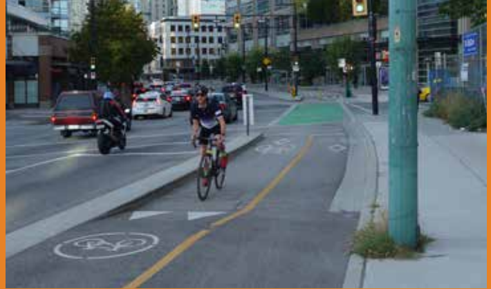
Separated bike lane installed on busy arterial road
