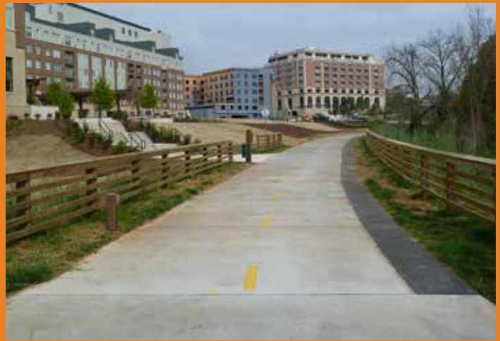
Infill development served by a regional trail
