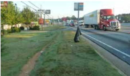
Pedestrian demand is shown by well-worn paths in the grass. Incomplete and hazardous crosswalks discourage compliance.
