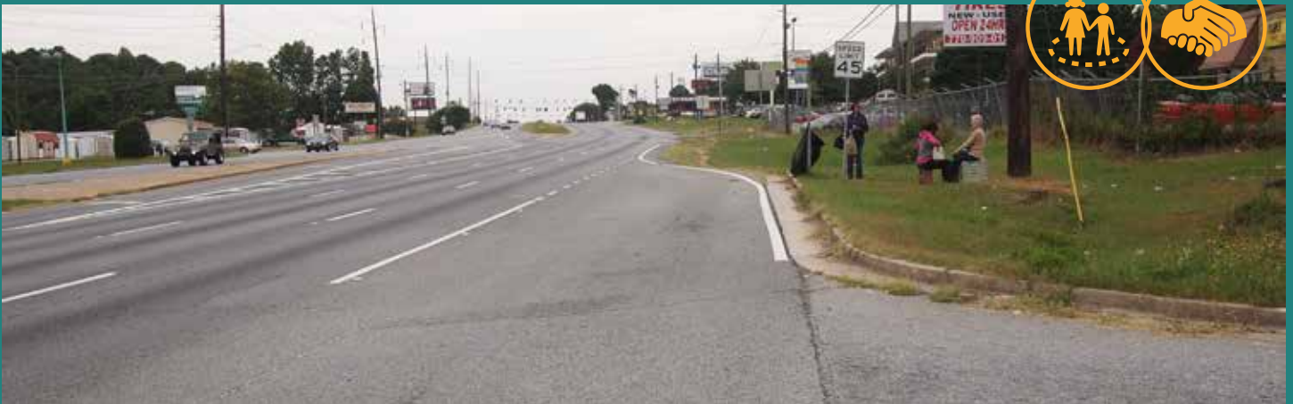
Transit users waiting at a bus stop with no sidewalk, crosswalk, seating or shelter.
