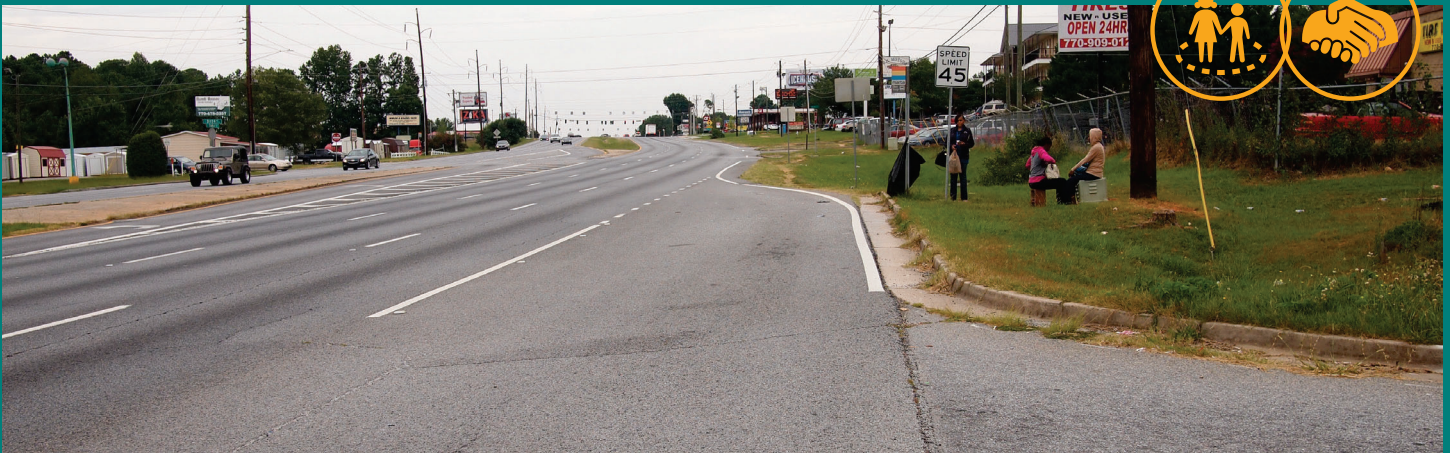
Transit users waiting at a bus stop with no sidewalk, crosswalk, seating or shelter.
