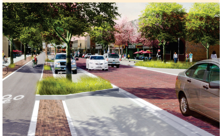
Before and after, Complete Street example in downtown Denison, Texas.
