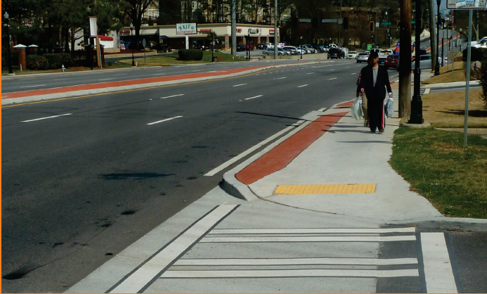
Basic sidewalk infrastructure on major road
