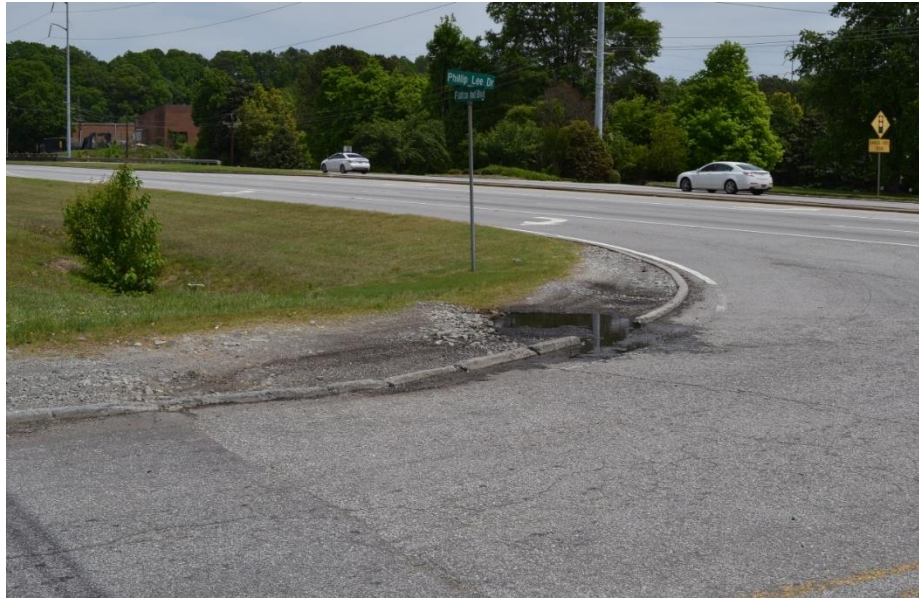
Figure 34: Curb Cracking and Off-Road Rutting at Intersection of SR 70/Fulton Industrial Boulevard & Phillip Lee Drive
