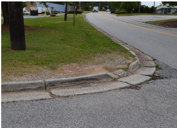
Figure 3. Cracked Curb and Off-Road Rutting
