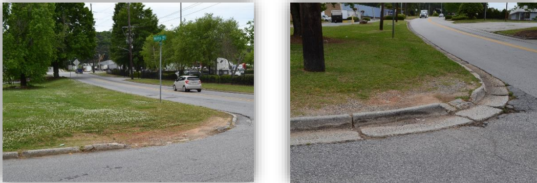
Figure 1-6. Curb Rutting at Patton Drive/Mills Place (Left) and Curb Cracking at Wendell Drive/Interchange Drive (Right)
